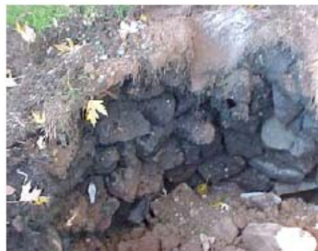
Figure 5. Collapsed Cesspool
