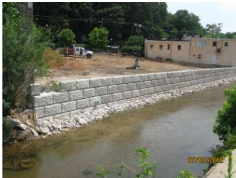
Codorus Creek Urban Streambank Stabilization
