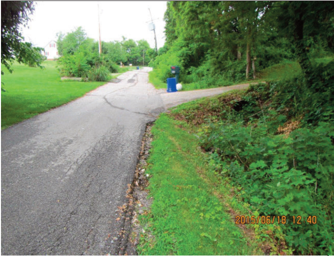
Church Avenue Before (Felton Borough)
