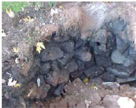
**Figure 4. Collapsed Cesspool**
