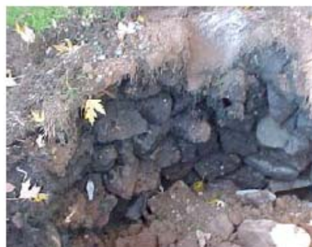
Figure 5. Collapsed Cesspool
