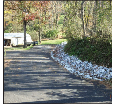
Above Photos: Eroded ditch at end of road that outlets to stream (left); Looking down out-sloped road (center); Roadside ditch stabilized with rip-rap.
