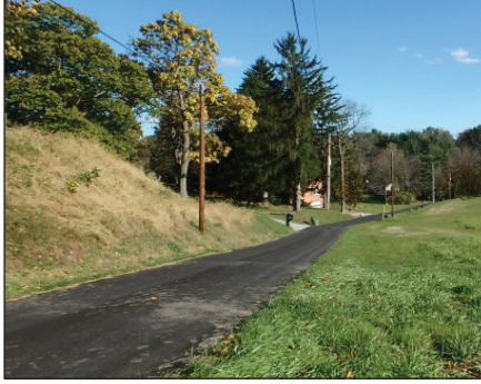
Above Photos: Eroded ditch at end of road that outlets to stream (left); Looking down out-sloped road (center); Roadside ditch stabilized with rip-rap.
