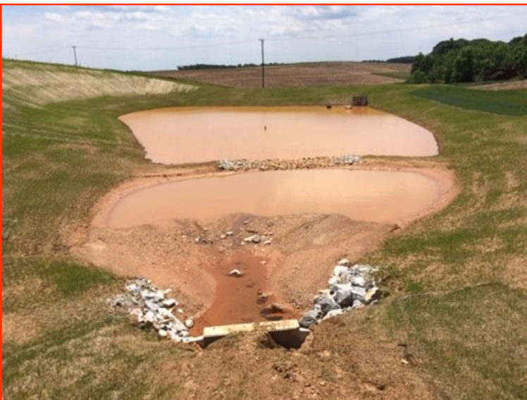
Above: Skimmer sediment basin with forebay capturing sediment from a residential subdivision under construc-
