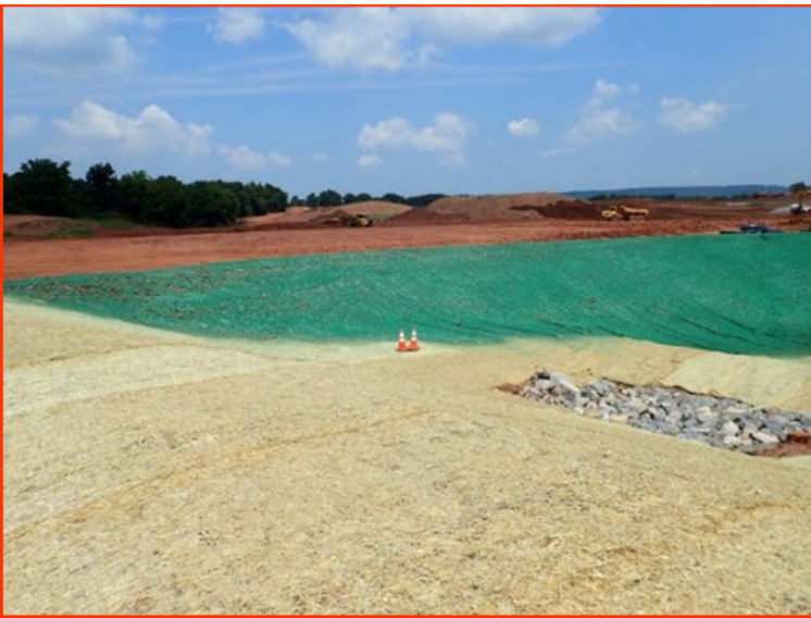
Above: Steep slope has been hydro-seeded and mulched.
