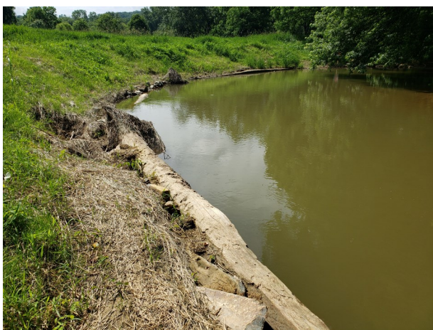
Mudsill Cribbing Best Management Practice for Stream Bank Protection
