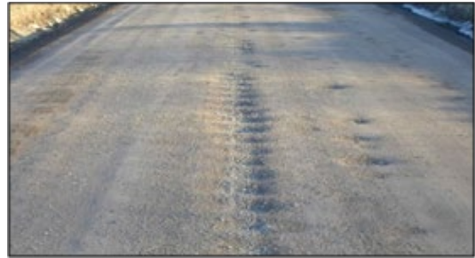
Figure 20. Potholes.
