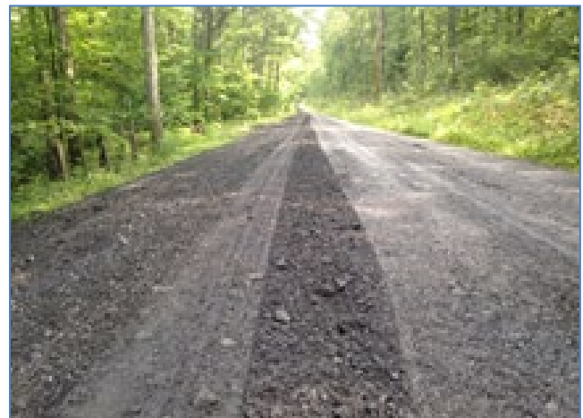
Figure 32. Before & after first pass of 10-ton roller.
