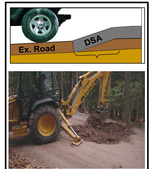
Figure 11. Paving Notch cut across road to support end of placement.
