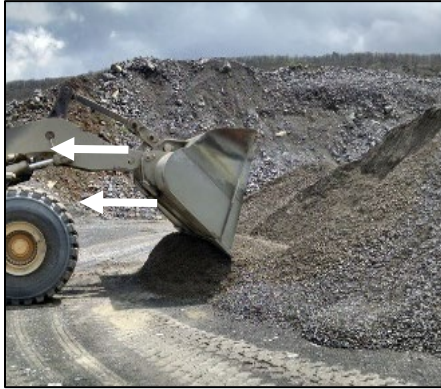
Figure 3. Forming the pad
