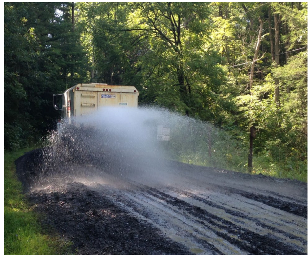
Figure 27. Adding water to a dry road surface.
