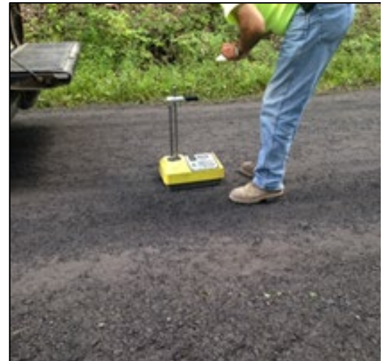
Figure 17. Compaction Testing with Nuclear Density Gauge
