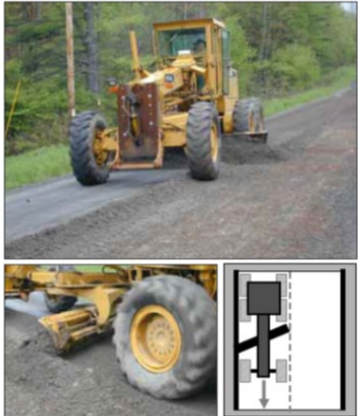
Figure 28. Place grader on one side of crown for each pass.
