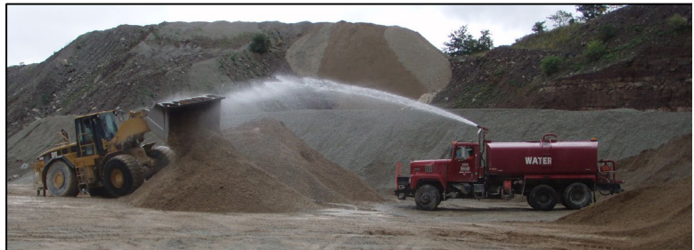
Figure 8. Mixing and adding moisture to a small DSA pile at a quarry.
