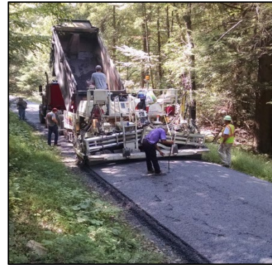
Paver placement of DSA.
