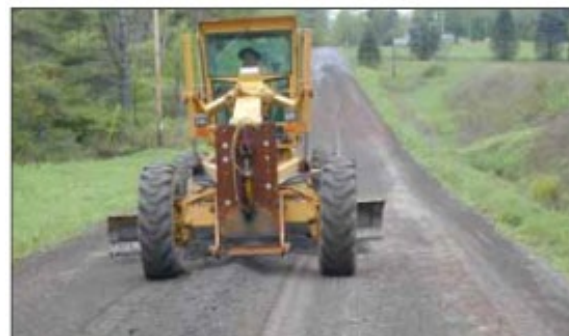
Figure 29. Material is knocked down
