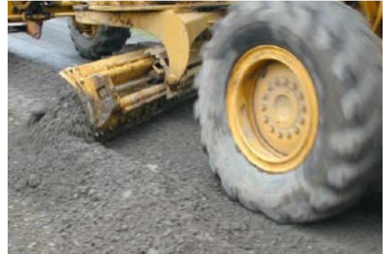
Figure 24: Wet material rolling off blade.
