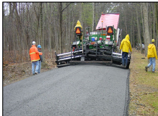
Figure 15. Paver placement of DSA with proper crown.
