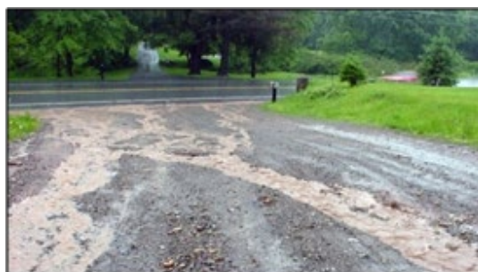
Figure 19. Water in wheel tracks.
