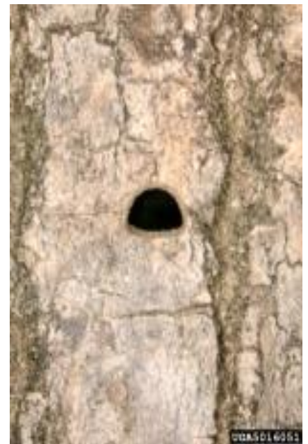
“D” exit holes
