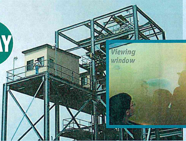
At left, water from above the dam attracts fish into the fish lift. A gate closes and crowds the fish over a bucket, which lifts the fish, in water, and releases them into the channel at a level above the dam.
