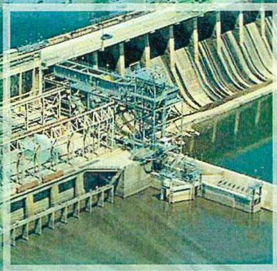
Conowingo Dam photos-PECO Energy
