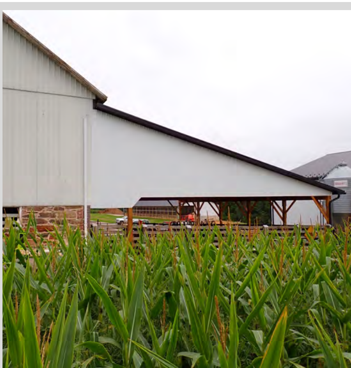
Above: Barnyard runoff problems are common across the county. To protect pastures during inclement weather, animals are often confined and fed in barnyards. Stormwater that falls on the barnyard comeslingles with manure and exits the barnyard. This contaminated stormwater must be managed. One solution is to eliminate stormwater from entering the barnyard by installing a roof over the barnyard. The roofed barnyard pictured was cost-shared by ACAP.
